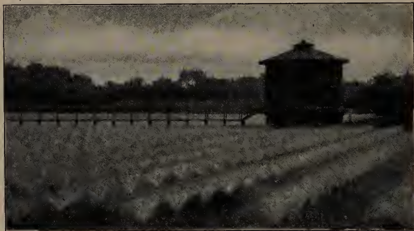
FIG. 13. Sewage-disposal plant at Columbus, Ohio, in which the sewage is sprayed into the air to secure its oxidation
